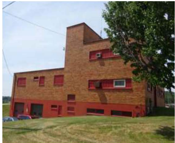
Rear Facing SW
