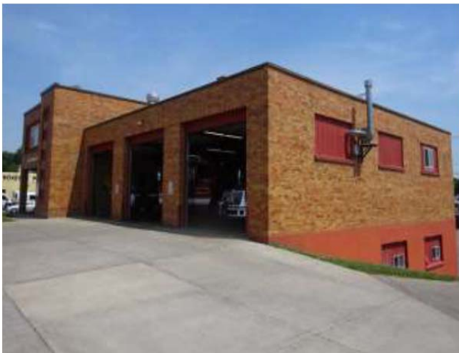
Front Facing SE
