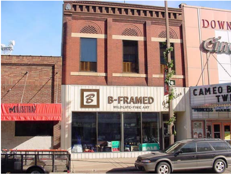
Good example of intact cornice
