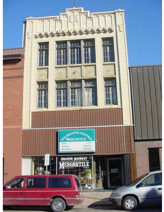
Well-maintained upper façade
